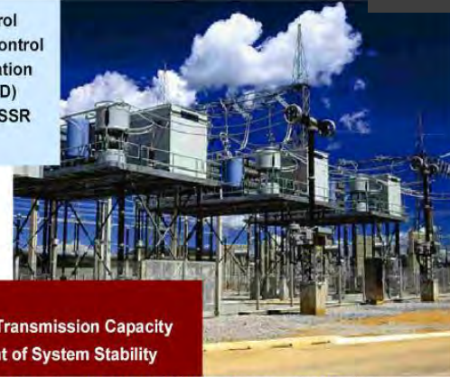
Fig. 7: TCSC in Brazil: 500 kV AC Long Distance Transmission
