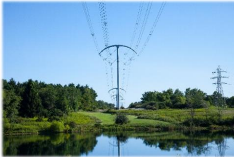
345kV BOLD Double-circuit (3-conductor)
